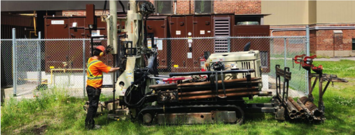
Figure 27: Borehole drilling equipment.
