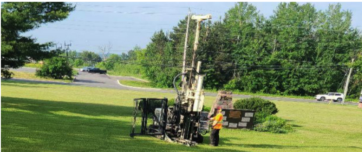
Figure 26: Borehole Drilling in East Section.
