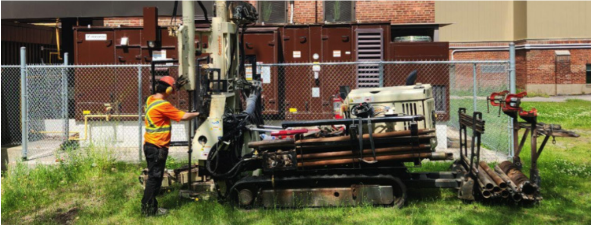
Figure 27: Borehole drilling equipment.
