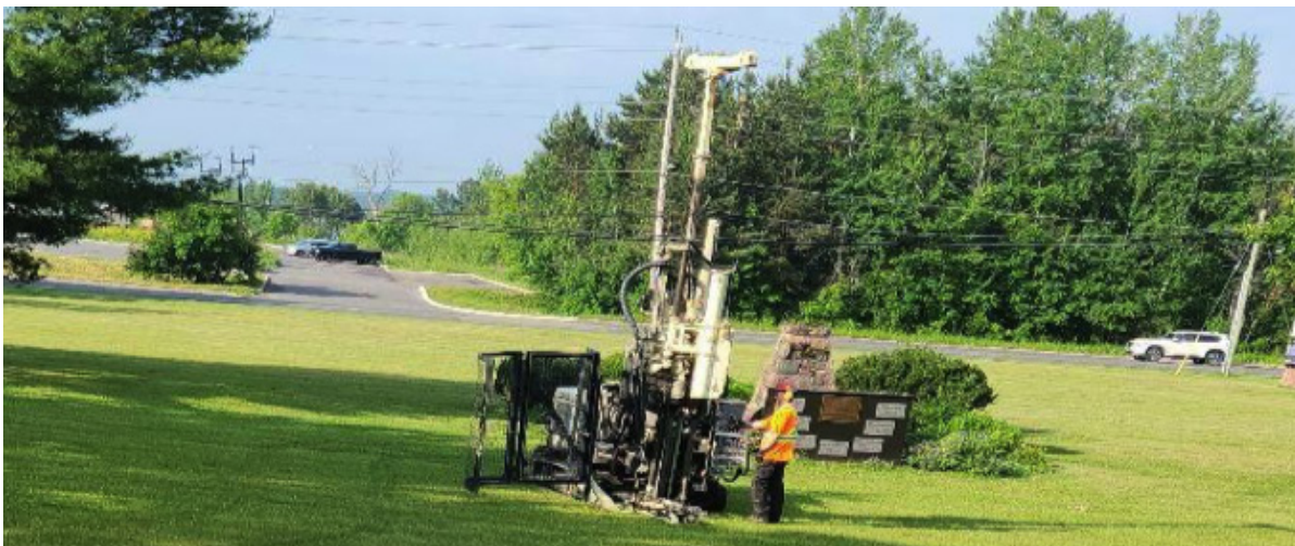
Figure 26: Borehole Drilling in East Section.
